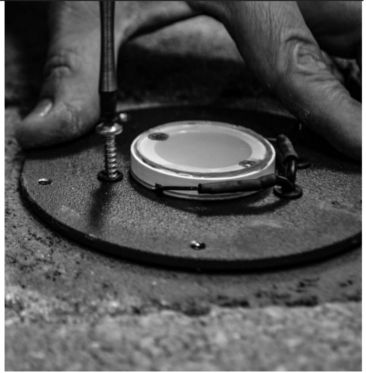
6. Attach fixture back plate to the surface using the previously drilled mounting holes. Note: We recommend using silicon to seal the back plate to the surface
