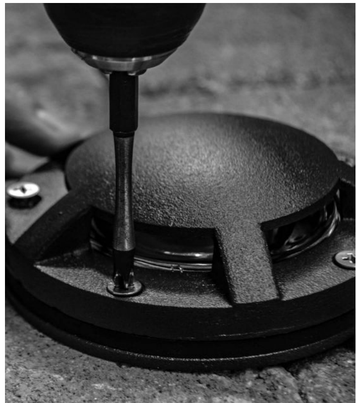
4. Remove Back plate from fixture
