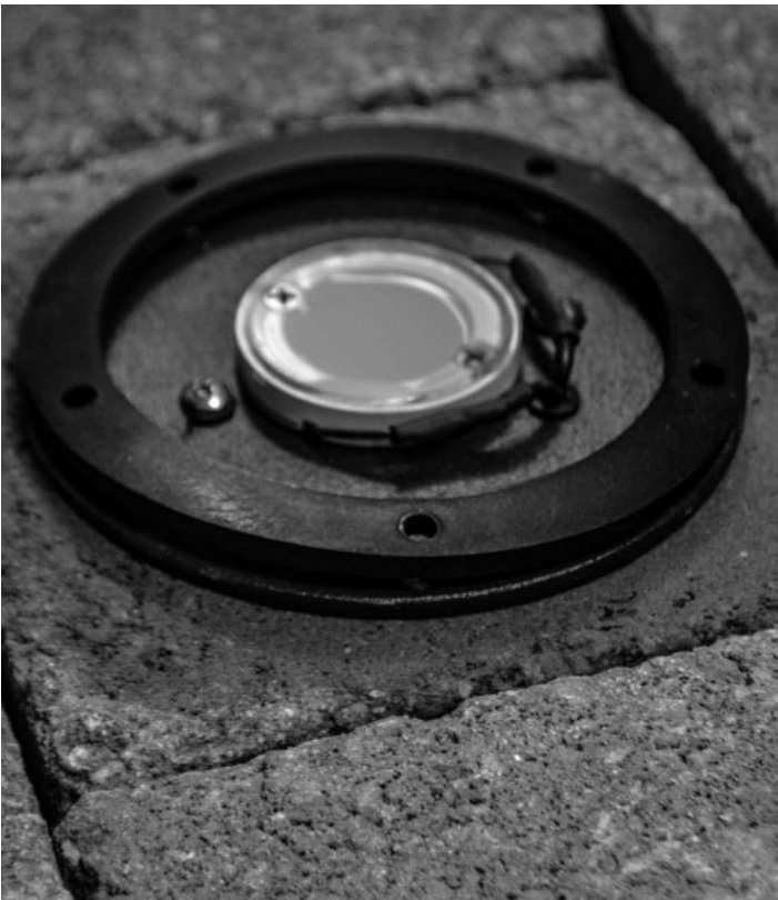
7. Place the gasket on the mounting plate
