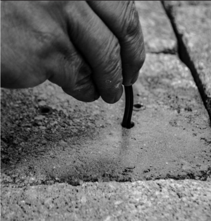
5. Feed wire through wire hole
