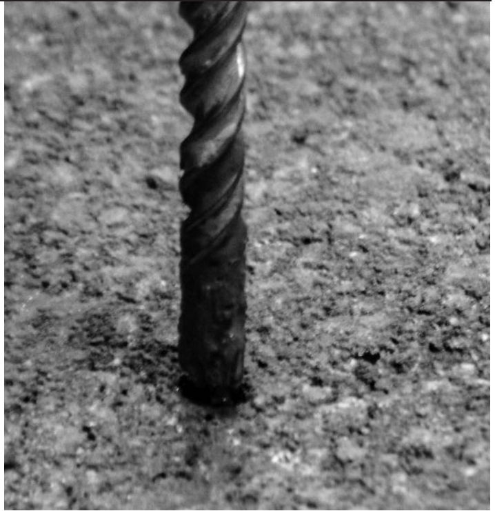
2. Drill three 1/4" holes using a masonry drill bit
