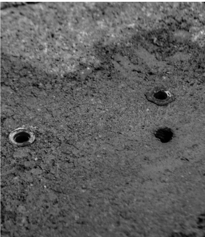
3. Insert anchor bolts into the two mounting holes Note: Do not use anchor bolt in the wire through hole
