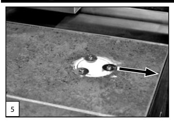
(5) Make sure to aim one of the screws towards the front of the counter. The front of the Quick Connect base will face this direction. Allow maximum drying time as specified by adhesive manufacturer.
