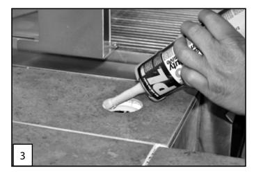
(3) Apply adhesive into hole. Make sure the adhesive is applied to the entire wall of the hole.
