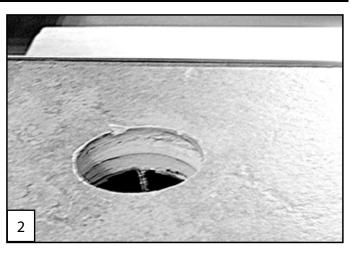
(2) Clean and dry hole prior to next step. Walls of hole should be free of dust, debris and moisture.
