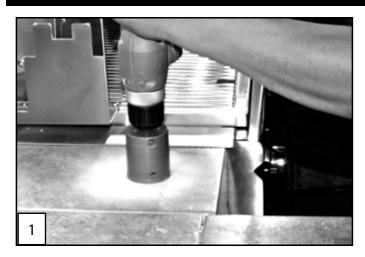
(1) Drill 2" hole through surface. A wet drill is recommended for hardscape installs. CAUTION: Make sure area underneath is clear of wire, conduit, gas lines, etc.
