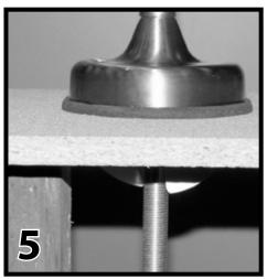
Tighten white butterfly nut onto threaded nipple until fixture is secure.
